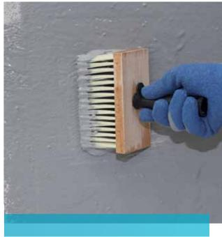
ELOTEX® redispersible polymer powders facilitate the application of flexible waterproofing membranes on substrates which are difficult to coat. The resulting polymer-modified membrane is resistant against chloride and sulphate ions, CO<sub>2</sub> and other aggressive media.
