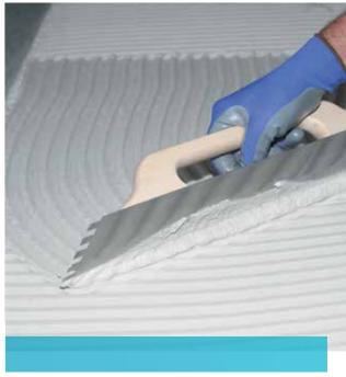
ELOTEX® and BERMOCOLL® products for tile adhesives deliver high adhesive strength, high sag resistance, increased freeze-thaw stability and very good working properties.
